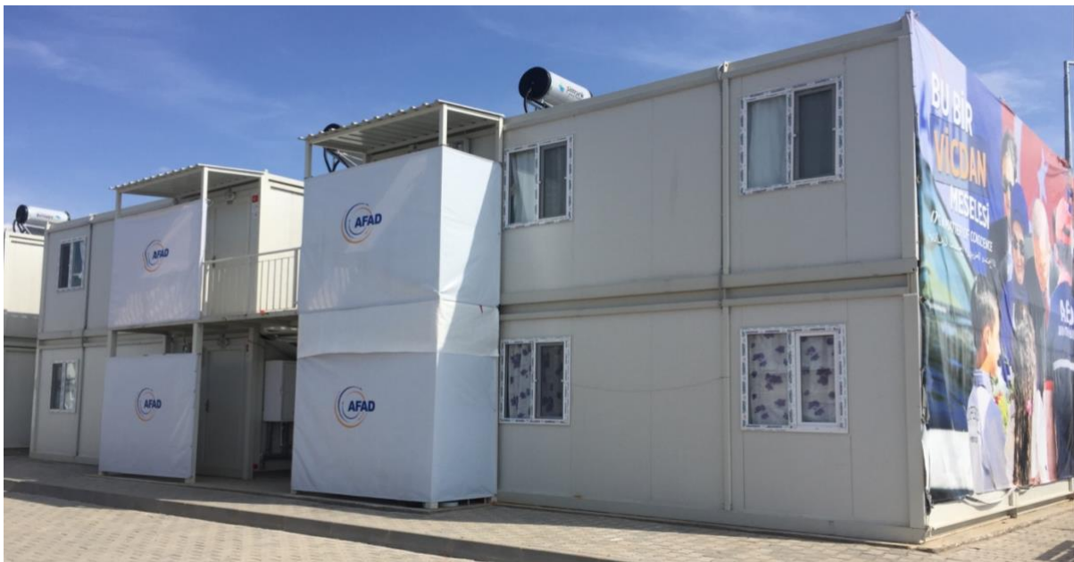
-Container Group where the combi boiler is installed (8 containers)
