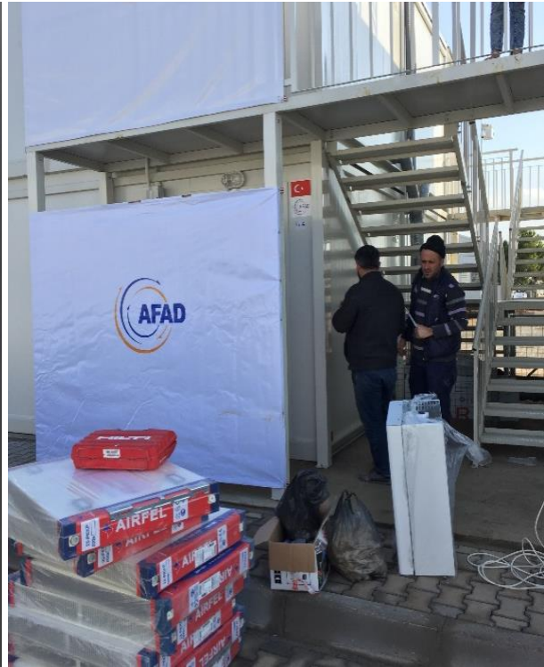
Installation to the Container
