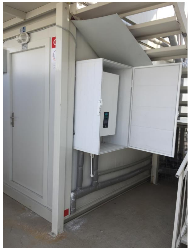
-Combi Boiler Installed
