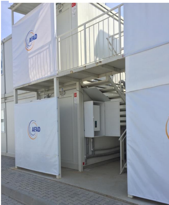
-Combi Boiler Installed
